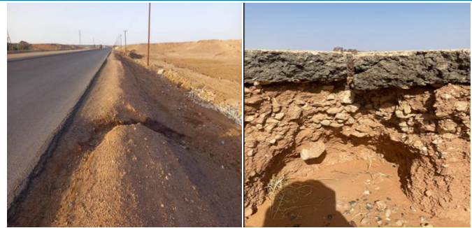
Fig.6: Shoulders Erosion
