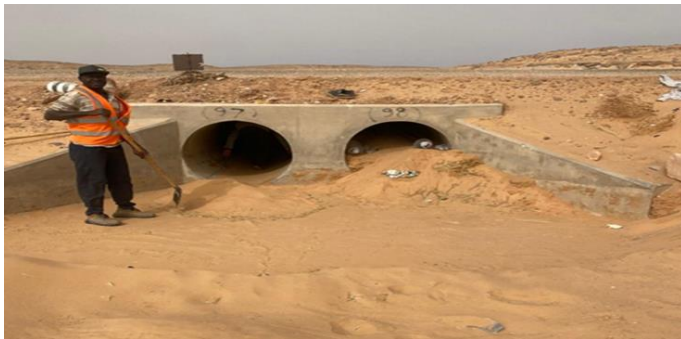
Fig.8: Blocked Culverts
